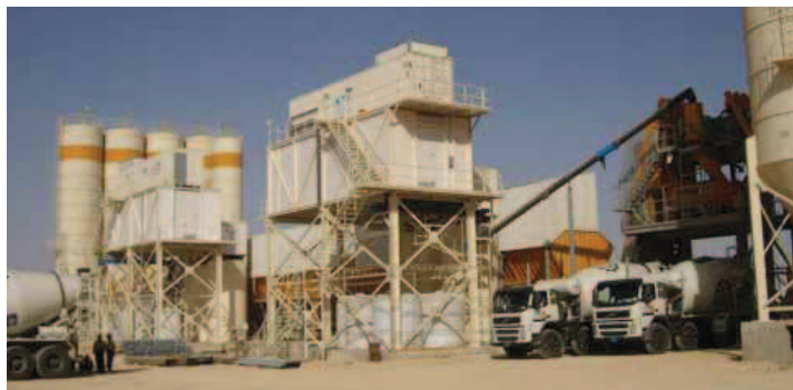
KTI Plersch is in the business of keeping concrete cool.
